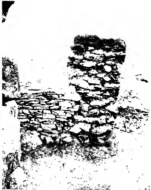
Fig. 206. Idalion. Wall 125 (left) and 19 E (right).
